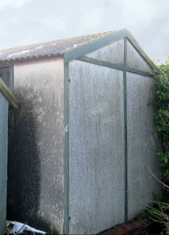
Asbestos cement panels and roof sheets
