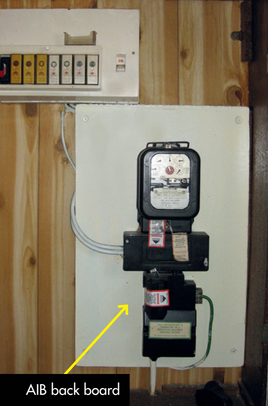
Asbestos flash guard
